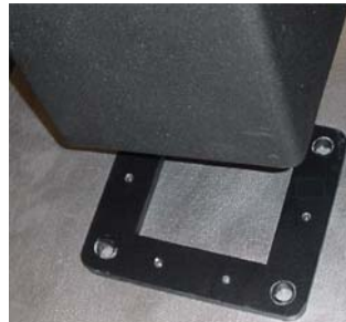
Figure 4 Setting the lower tower section down over the base plate.
