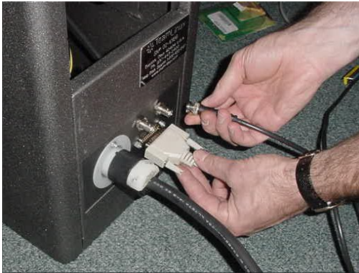
Figure 9 Connecting external cables for (left to right) power, serial communication, and video. Video In connection is not in use.
